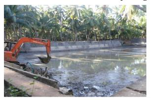
nylon wastes and other rubbishes are removed. Algae and water weeds found inside the open wells are removed completely. Silts formed over the bed of the open wells which are sedimentation of sand particles over the years are carefully removed. Steel cover with opening facilities on both sides is fitted on the top of the open wells. Circular parapet walls of the open wells are cleaned and painted.
